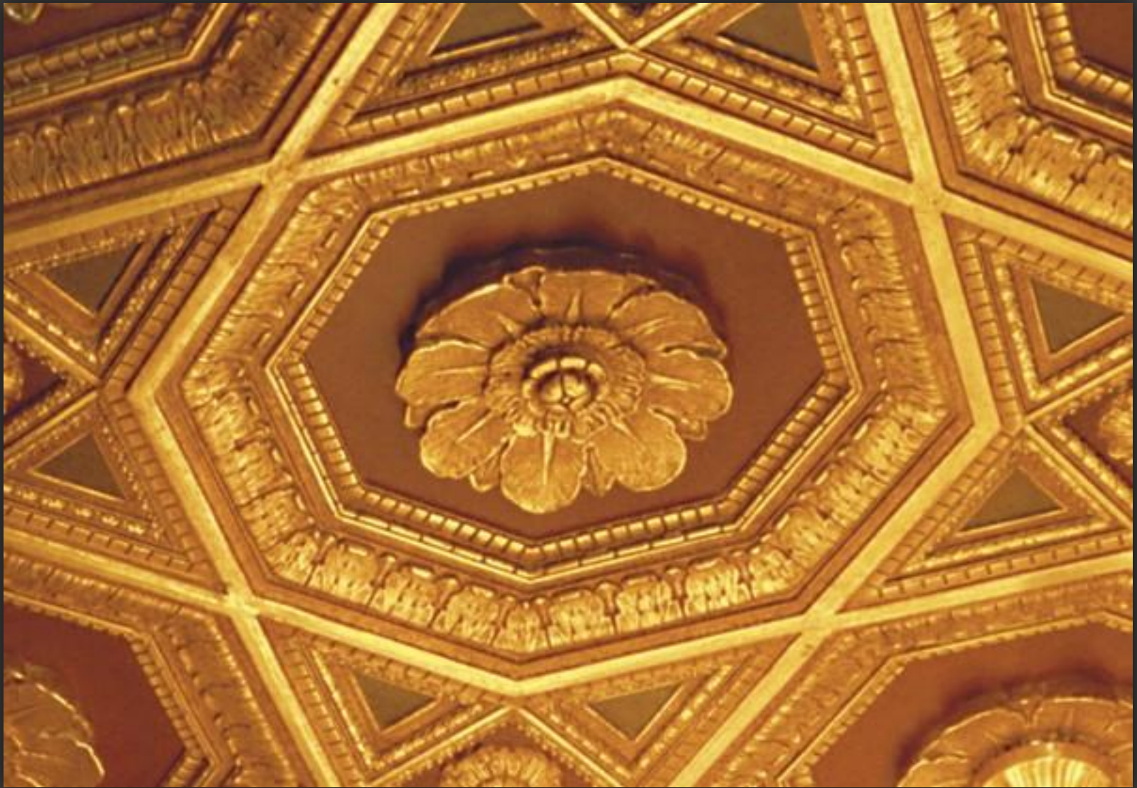
Interior restoration – Coffered Ceiling, 35 East Wacker, Chicago, Illinois
