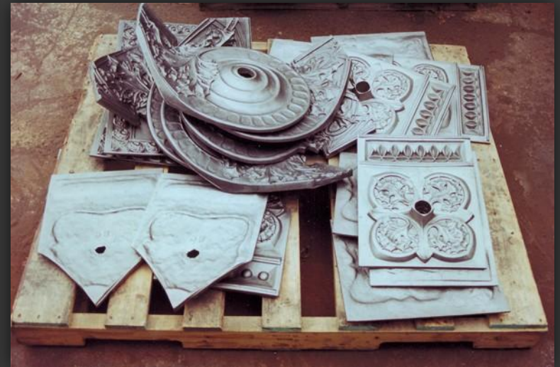
Interior restoration and recreation of forged iron light fixtures – Ganz Hall. Roosevelt University , Chicago, Illinois
